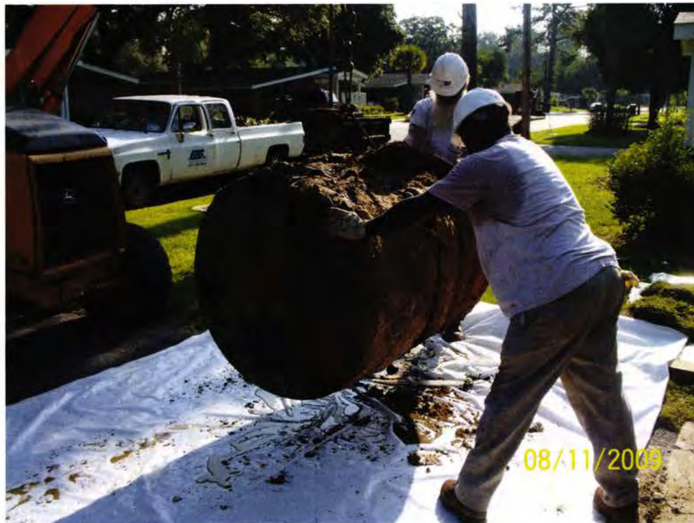
Picture 2: UST 1469Cardinal removal in progress.
